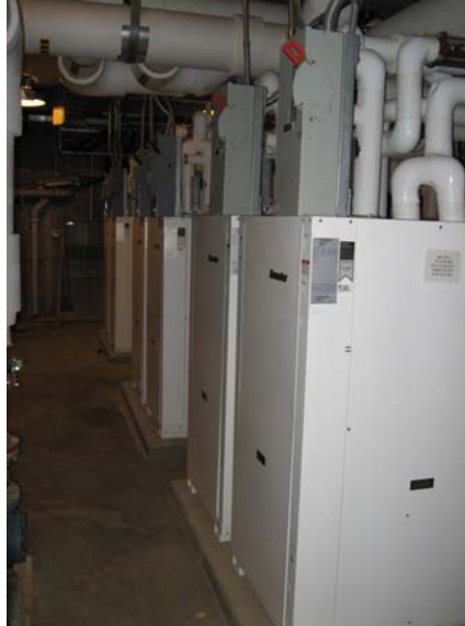
CSI's original heating and cooling system has been expanded to accommodate more buildings since its installation in 1979. (Randy Dill/ College of Southern Idaho)
